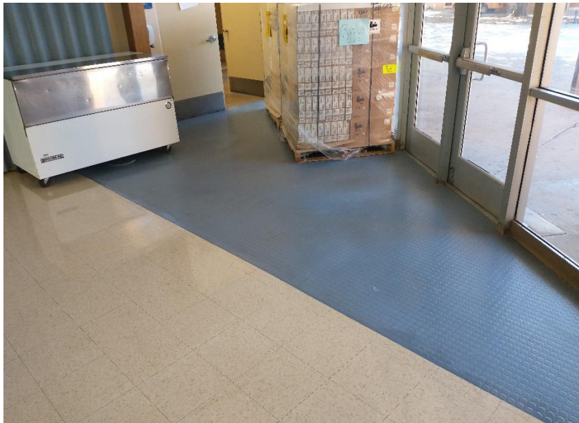
Main cafeteria – 12" vinyl floor tile, blue rubberized entry flooring
