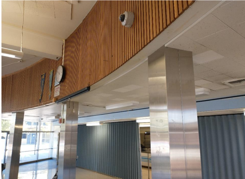
Main cafeteria – Varnished wood slat decorative wall treatment, sheet metal covered columns
