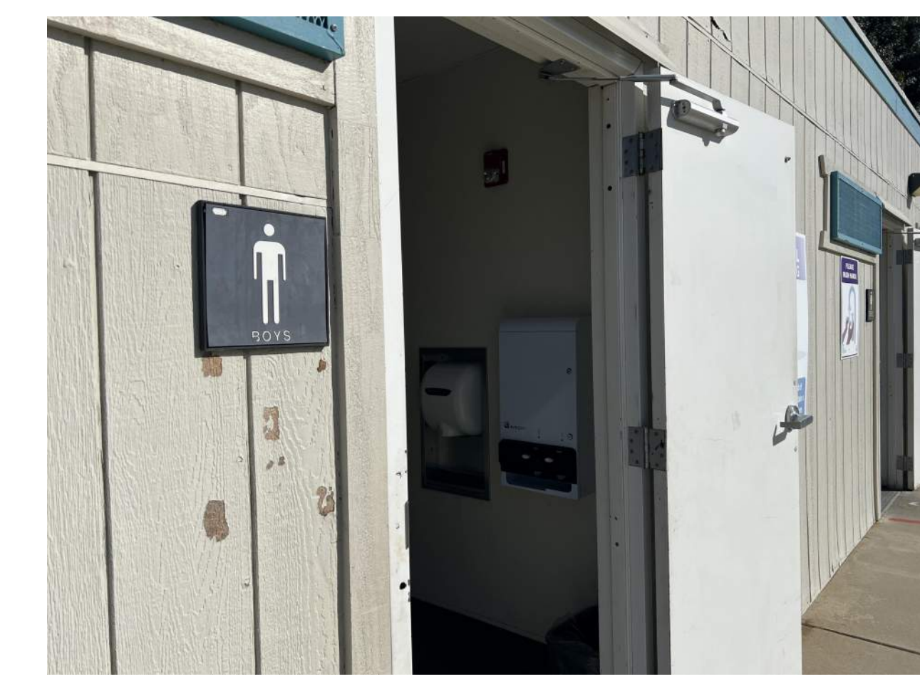
P-101 BOYS RESTROOM -D. FIELD VERIFIED CONDITIONS
