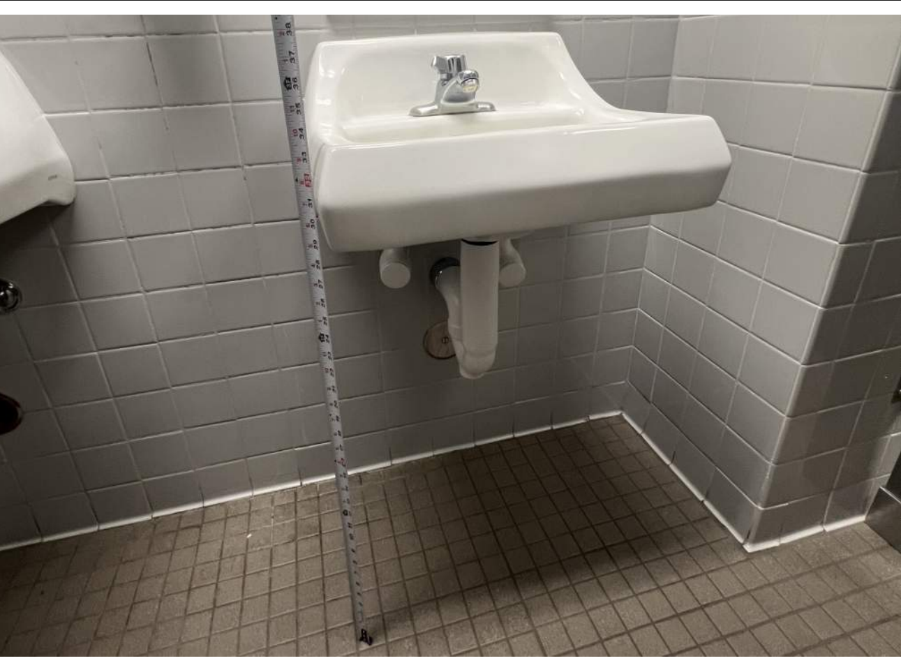
P-101 BOYS RESTROOM -E. FIELD VERIFIED CONDITIONS
