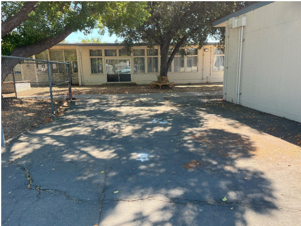
Photo No. 2 – CPT2 location in existing pavement facing south.
