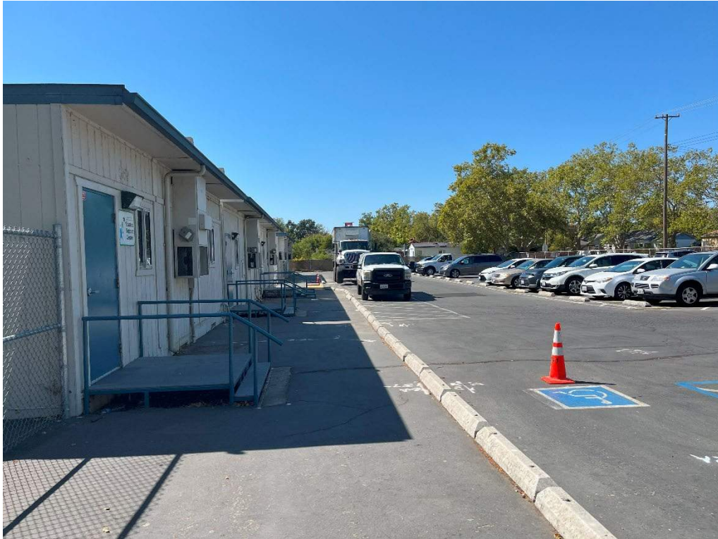
Photo No. 1 - Representative existing site conditions facing west.
