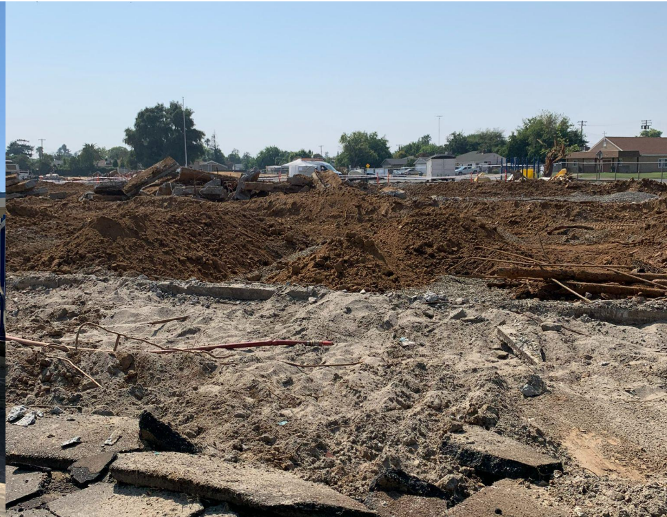
Old Nicholas is Demolished
